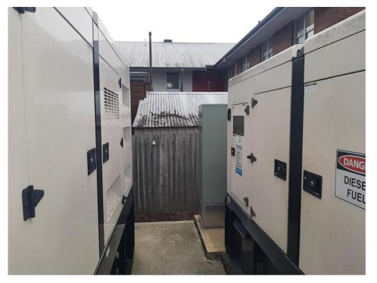
Figure 7 Existing 185kVA Genset (Right), Existing Spare 330kVA Unconnected Genset (Left) and MTS Transfer Switchboard (Behind)
