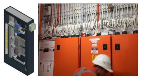
Figure 31 – Typical Distribution Board Cupboard
